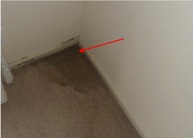
When the carpet is pulled back the water damage beneath is clearly visible – check for rust on carpet tacks
