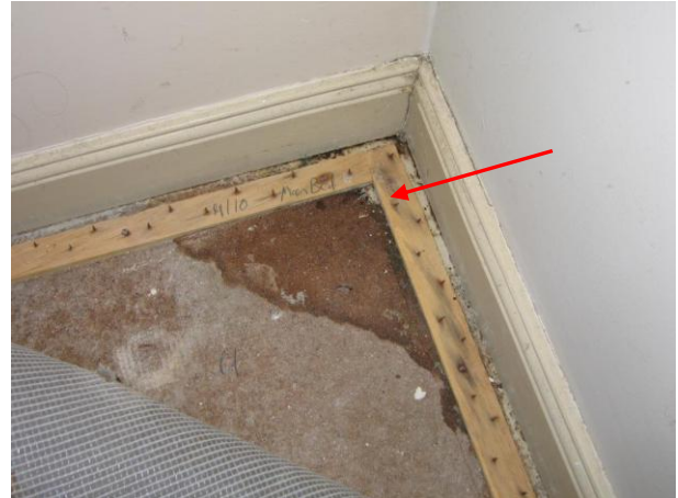
When the carpet is pulled back the water damage beneath is clearly visible – check for rust on carpet tacks
